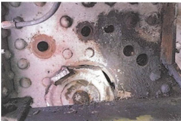
Photos of the river-side 2 nd Link Pin showing misalignment of bolt holes, missing bolts, and wear at the main pin.
