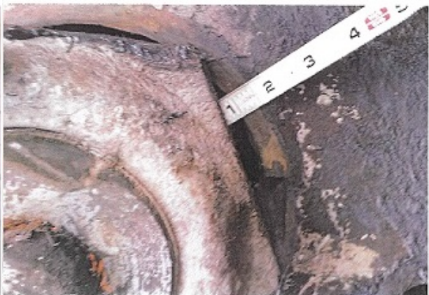
Photos of the river-side 2 nd Link Pin showing misalignment of bolt holes, missing bolts, and wear at the main pin.
