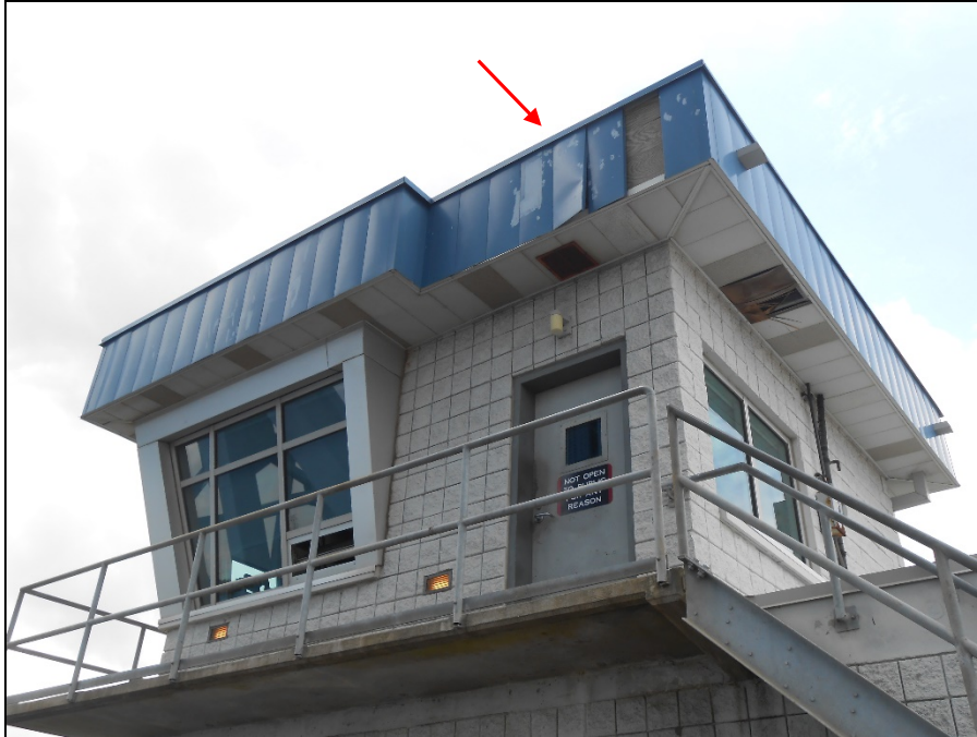
Photo shows damaged/missing roof fascia panels at the Bridge Operator's House.
