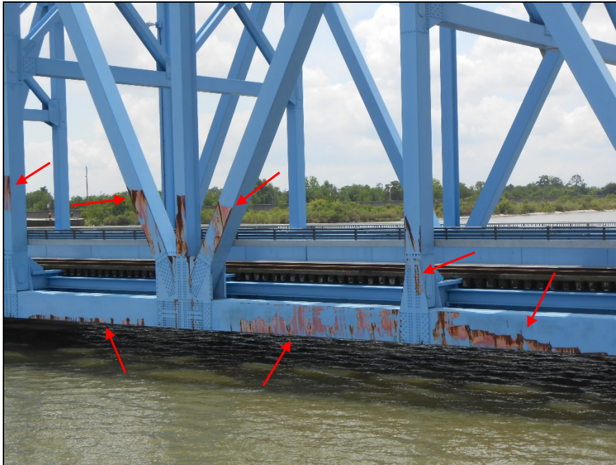
Photos show minor structural damage along the north side of the lift span.
