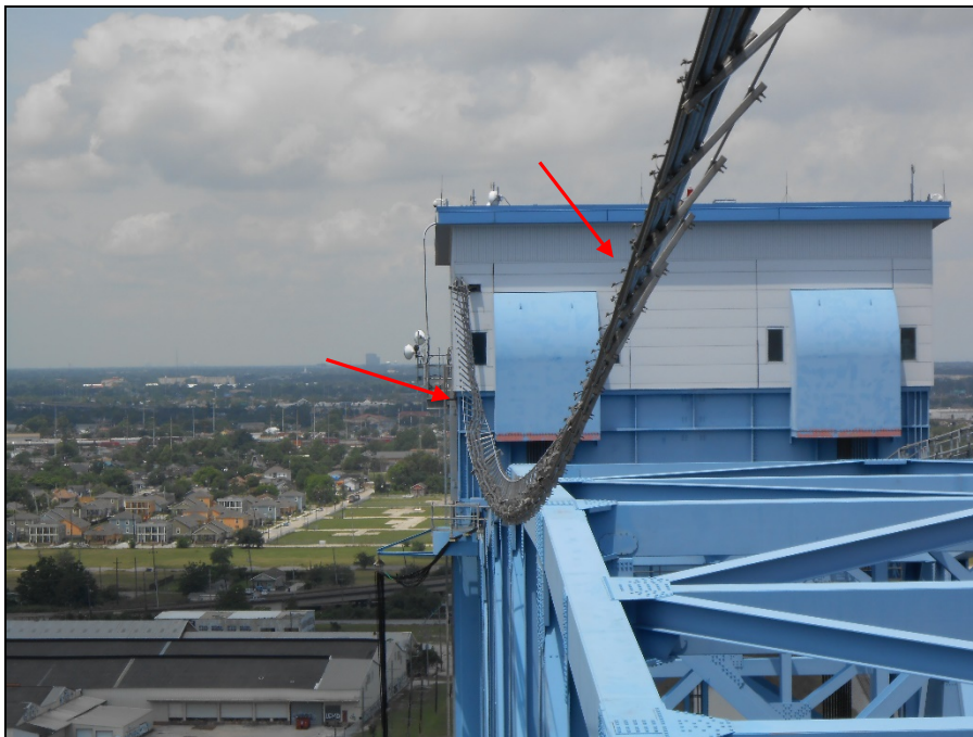
Photo shows misaligned/twisted aerial cable assembly.
